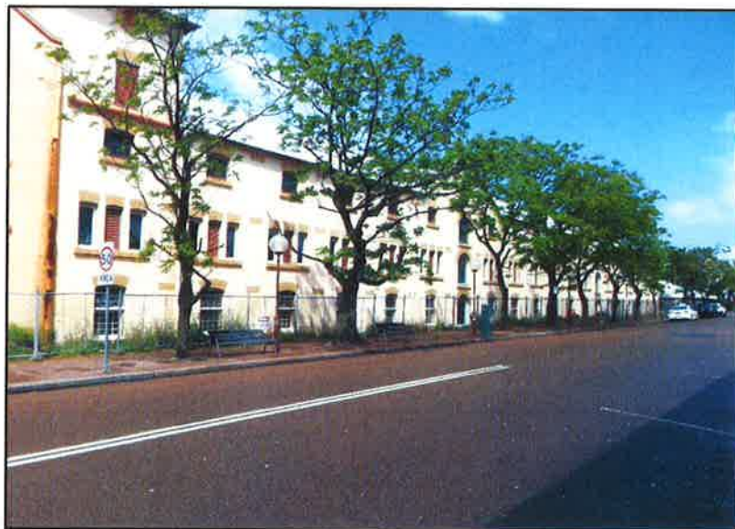
Photograph 8 – western edge of former Castlemaine Brewery site along Wood Street
