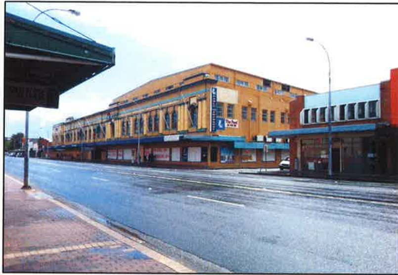
Photograph 7 – Local Heritage-listed former Newcastle Co-Operative Store diagonally opposite the site on Hunter Street
