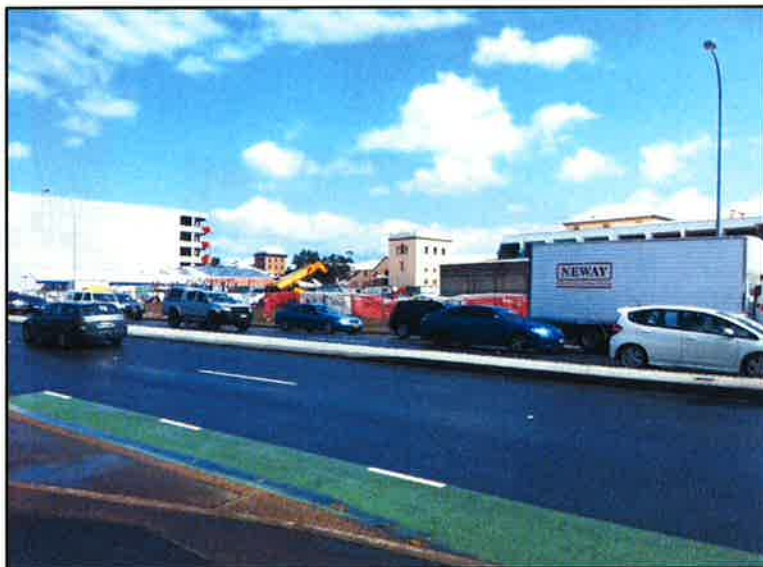
Photograph 2 –View north-west across the site towards new Gateway building
