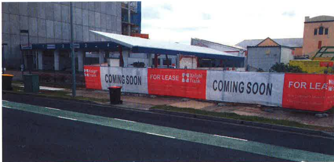
Photograph 1 – Proposed access location off Stewart Avenue.
