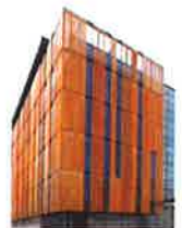
Example of façade with metal panels
